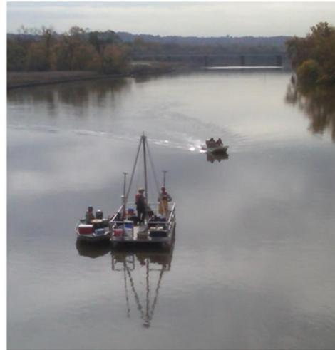
Boat-mounted drilling equipment was used to collect sediment samples from the bottom of the Anacostia River.
