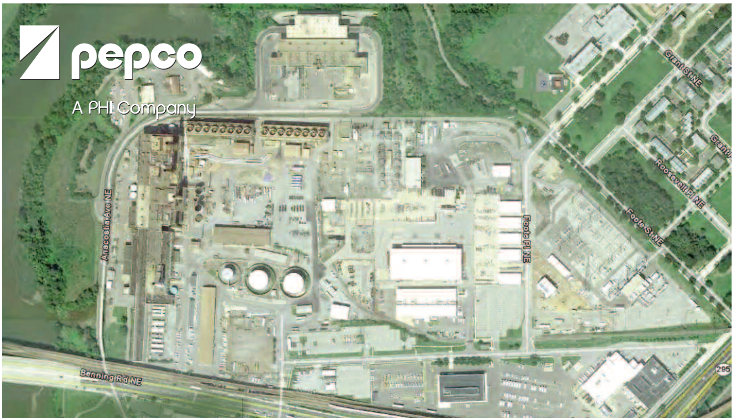
Aerial view of Pepco's Benning Road property.
