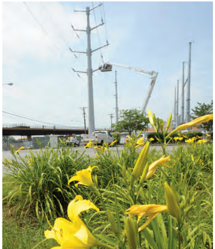
This rain garden is part of Pepco's low-impact development program of storm water management. The garden's natural filtration reduces any impact on the river.
