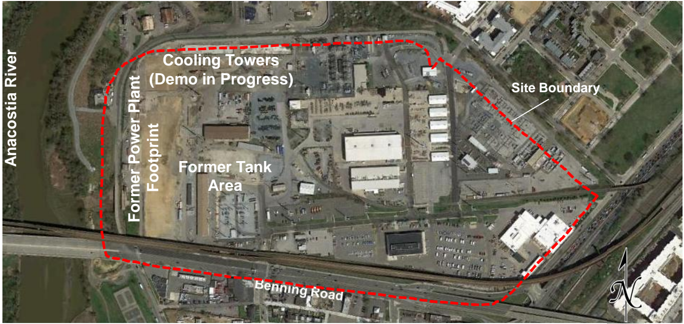
After Power Plant Demolition
